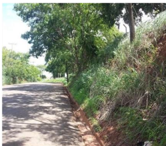
Figura 4. Talude 3 – Campus III da UNESP. Sanches (2015).
